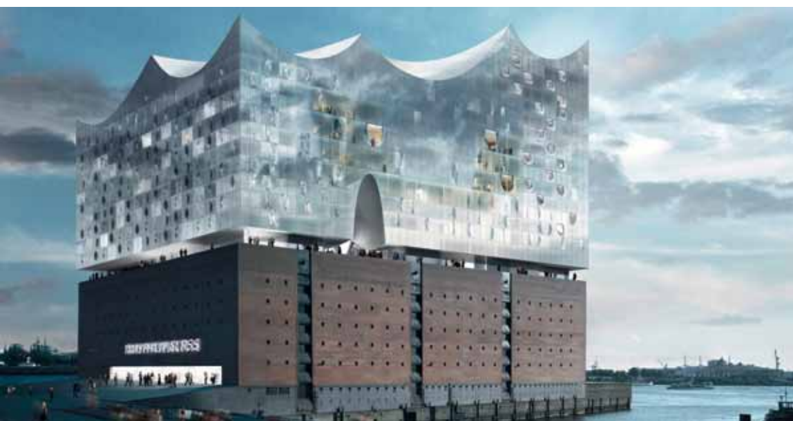
Elbphilharmonie under construction Architect: © Herzog & de Meuron, Basel (Switzerland)
