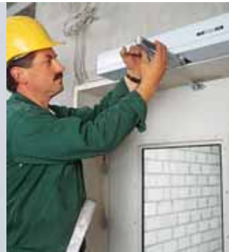
Specialist facility consulting
